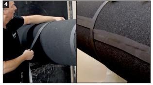
When mounting the Kaifsound sheets on pipes, the adhesive seam tape should additionally be secured by means of the use of Kaiflex tape. Furthermore, at least 3 additional Kaiflex tapes should be applied at right angles to the seam to secure it.
