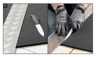
The Kaisound sheets must be cut with a very sharp knife. In order to be able to perform a straight cut, a metal guide rail should additionally be used when cutting the sheets.
