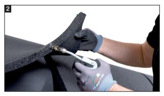
The Kaisound sheets are bonded together with the Kaiflex Special Adhesive 414. In doing so, the special adhesive should be applied evenly across the cut surfaces on both sides. The air-drying time must be strictly adhered to.
